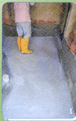
Substrate shall be flat and even
