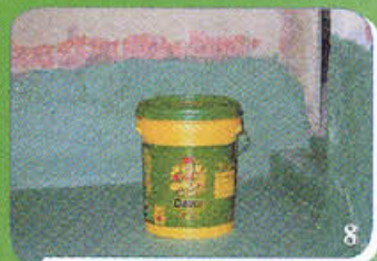
Completed 2nd coat
