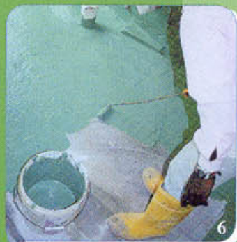
Apply one layer at a time using a mini lamb's wool roller
