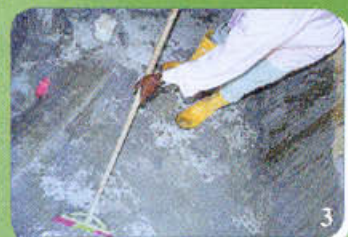
Water is evenly saturated using a brush
