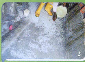
Substrate shall be visibly dry or dampened by sprinkling with clean water
